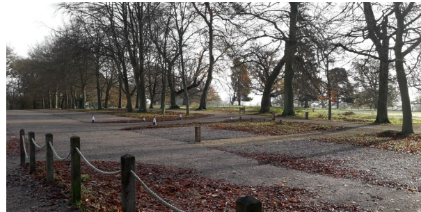
Image credit: The resurfaced gravel-filled Bodpave car park, and new grass-filled Bodpave overflow in the background, at Corfe Castle (photo by Imogen Wood).
