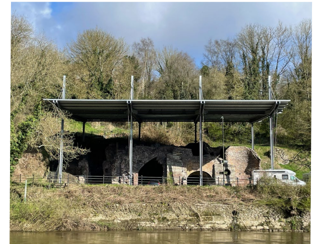
Image credit: The permanent shelter of the Bedlam Furnaces ruin in Ironbridge. Sites such as these, in the very long term, may be considered for adaptive release through allowing inevitable change to affect structural appearance and values contributing to significance. This applies particularly when external factors such as climate change cause greater impacts and make other adaptive strategies less tenable (photo by Imogen Wood).
